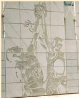
Kohl Center, University of Wisconsin. Precaster: Gate Precast Co. Photo: Steve Brock.
